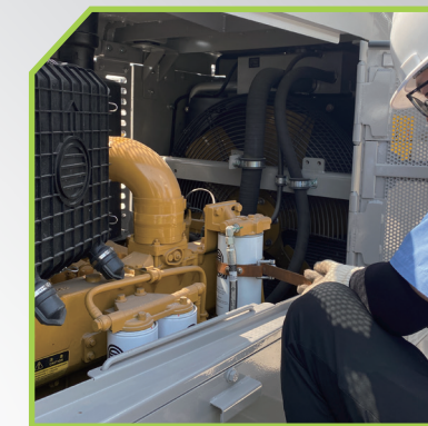
Fuel filter maintenance 燃油滤更换
