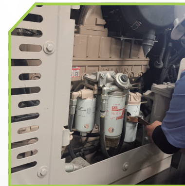
Oil filter maintenance 机油滤更换
