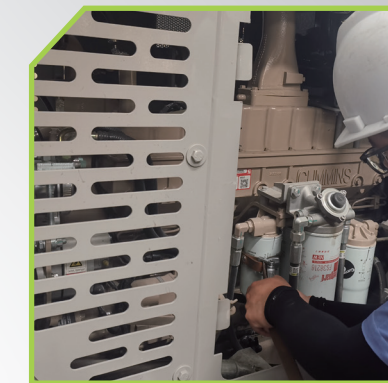
Fuel filter maintenance 燃油滤更换
